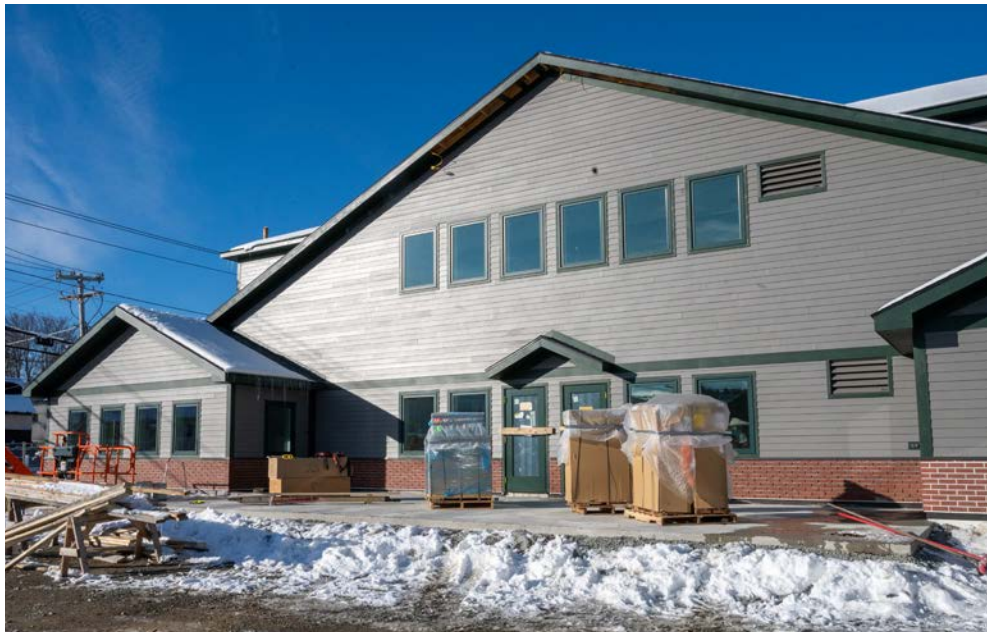
Construction progress at the Kogod Center in February 2024
