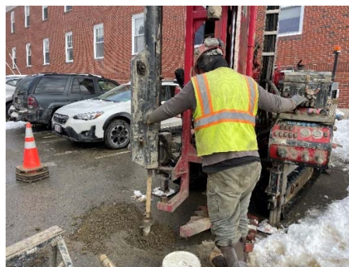
Sampling at Test Boring B-1
