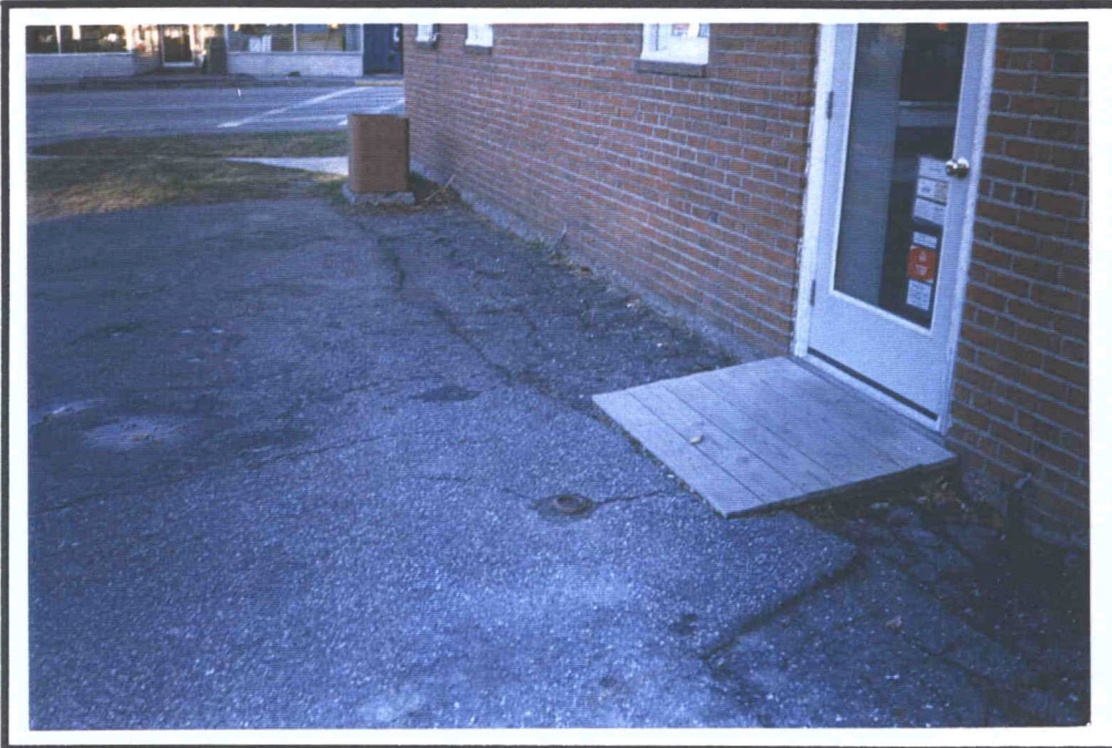
AREA OF THE TANKS PRIOR TO EXCAVATION. SHOWN IN THE PHOTO IS A FILL PIPE (IN FRONT OF THE DOOR) LATER DETERMINED TO BE CONNECTED TO A 1,000 GALLON TANK. IN THE BACKGROUND (AT THE BUILDING CORNER) IS A CONCRETE PAD LATER DETERMINED TO BE A PUMP ISLAND TO A 2,000 GALLON TANK.
