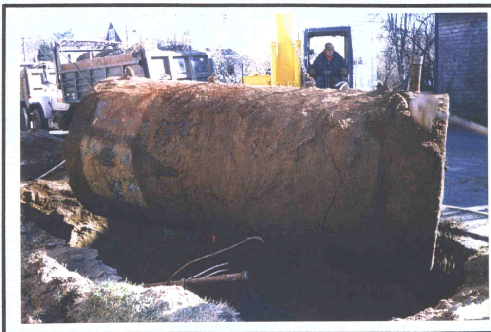
TANK #2, 2,000 GALLON TANK, DURING REMOVAL. SUCTION LINE TO A PUMP ISLAND IS VISIBLE IN THE FOREGROUND.
