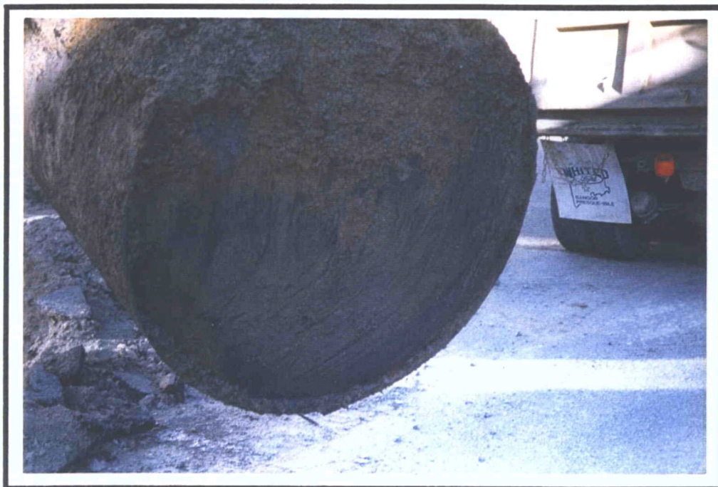
END OF TANK #1, 1,000 GALLON TANK, DURING REMOVAL. NOTE INDENTED SEAMS ON END OF TANK.
